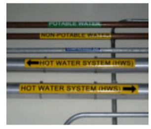
Colour coding of water pipes to avoid contamination
