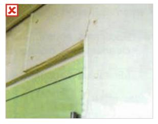
Cracks allow bacteria and molds to accumulate
