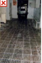
Floor with drainage of appropriate slope
