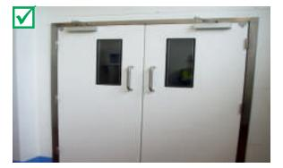
Doors made of smooth and non-absorbent surfaces
