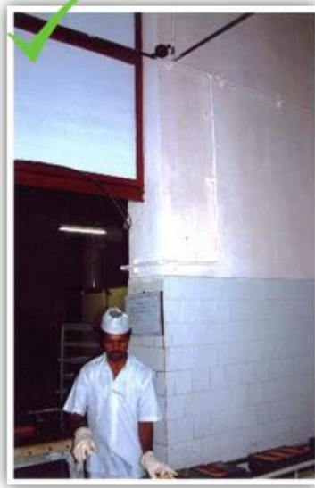
Good Repairs & Clean walls
