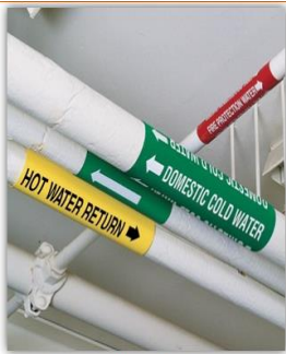
Colour coding of water pipes to avoid contamination
