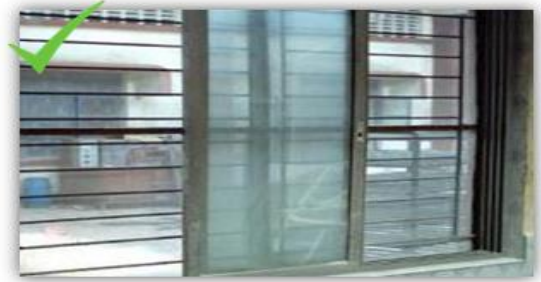
Well screened windows
