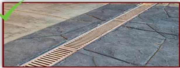
Floor with proper drainage
