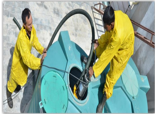
Cleaning of water storage tanks
