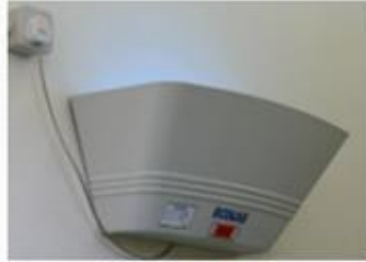
•Glueboard for insect trapping in production •maintain 1.5m radius gap
