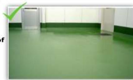
**Floor with drainage of appropriate slope**
