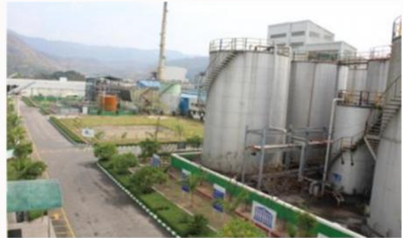
Demarcation of the area
