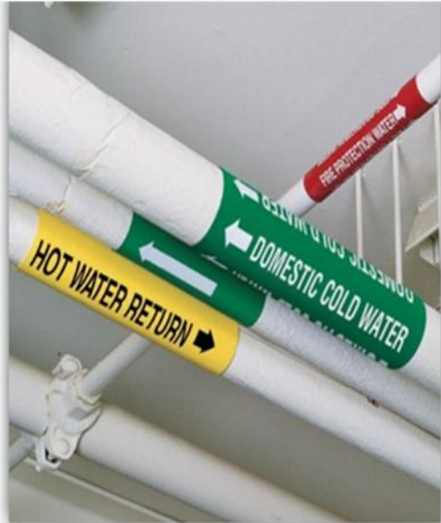
Colour coding of water pipes to avoid contamination
