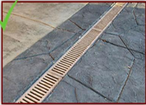
Floor with proper drainage
