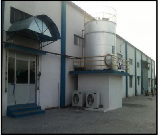
Pavers block in the premises
