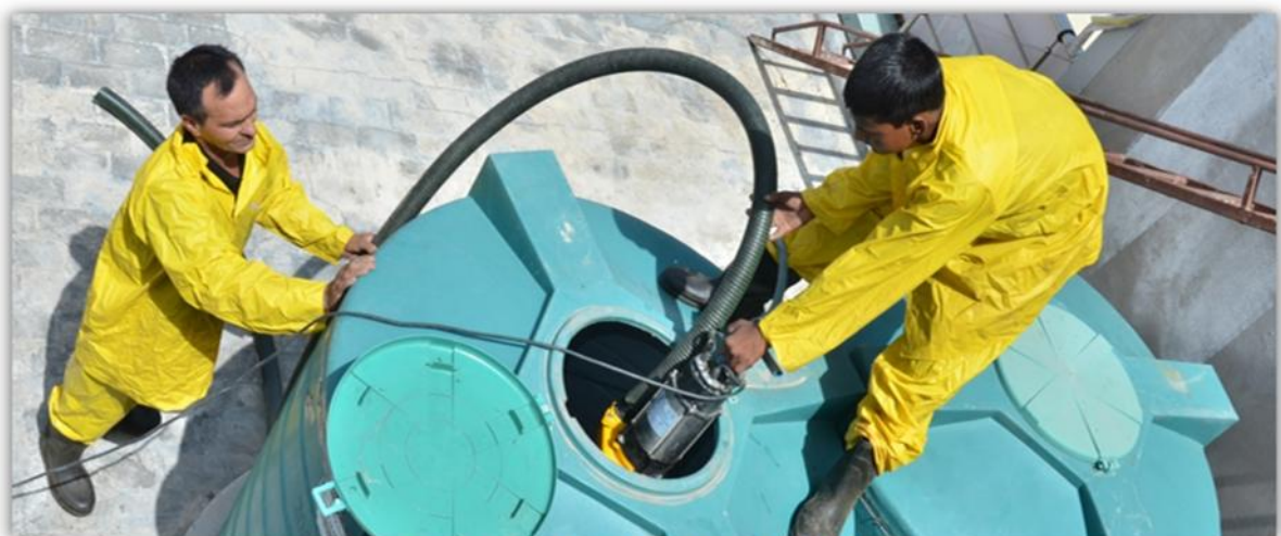
Cleaning of water storage tanks
