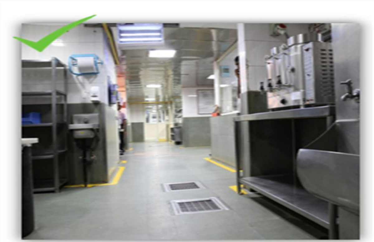
Drains should be covered to prevent insects and rodents
