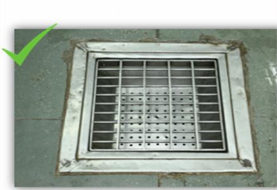
Drains should be covered to prevent insects and rodents
